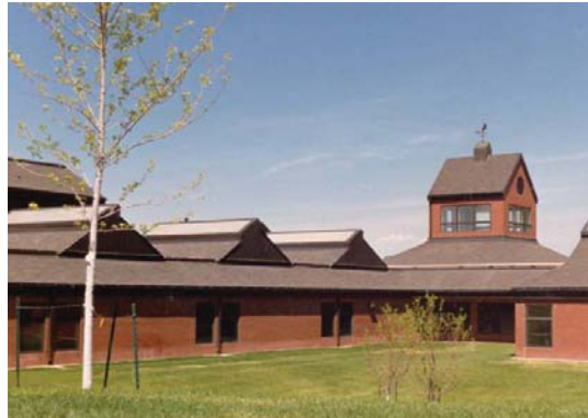
First fully-daylighted elementary school in 1985.
